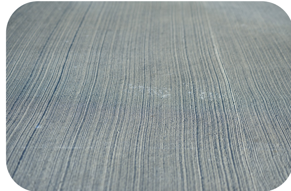
A nonslip concrete surface
