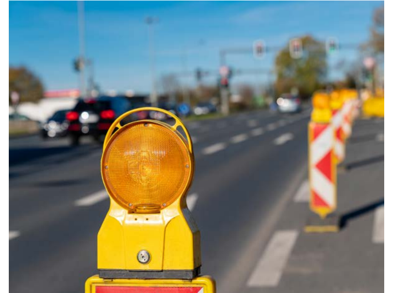
Conduct final sweep of site with photo verification
