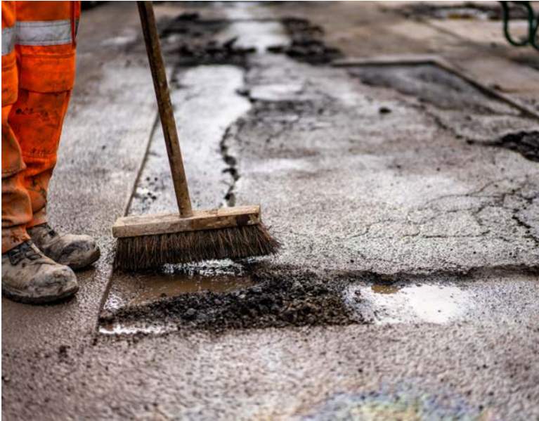
Remove trash and debris from performed work
